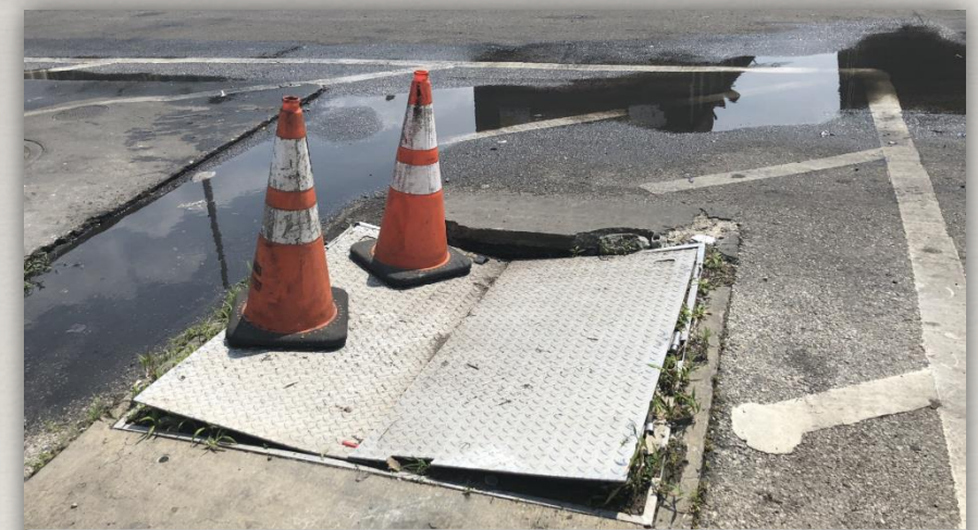
Underground storage cover is damaged
