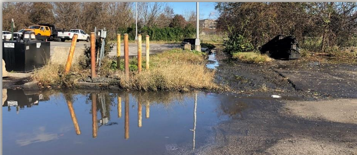
Unevenly graded parking lot results in icy road conditions
